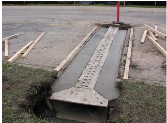
ACO ecopassage construction Photo provided by Parks Canada
